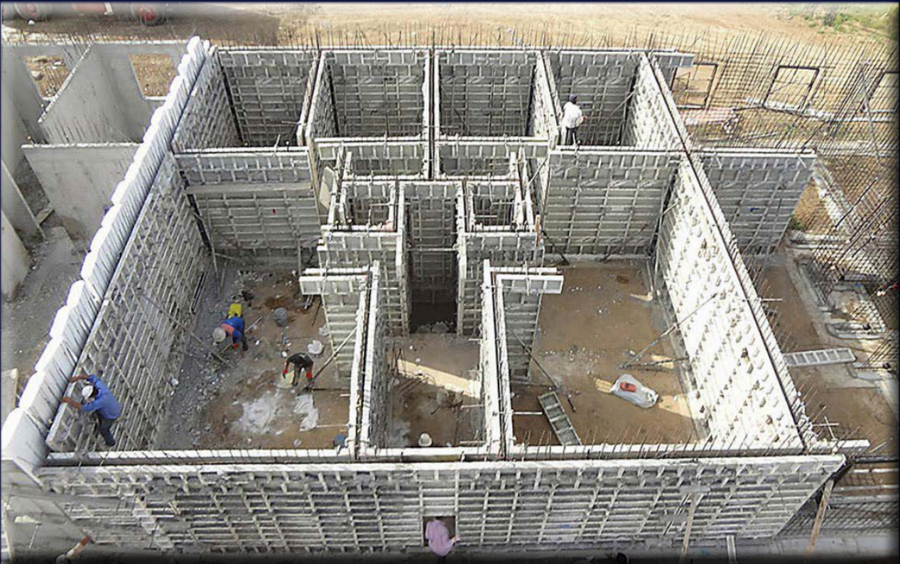
PRACTICAL APPLICATION OF ALUMINIUM FORMWORK SYSTEM
