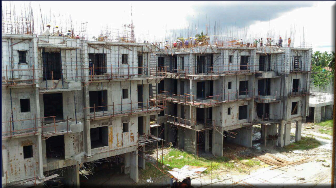
CONSTRUCTION SITE OF ALUMINIUM FORMWORK SYSTEM
